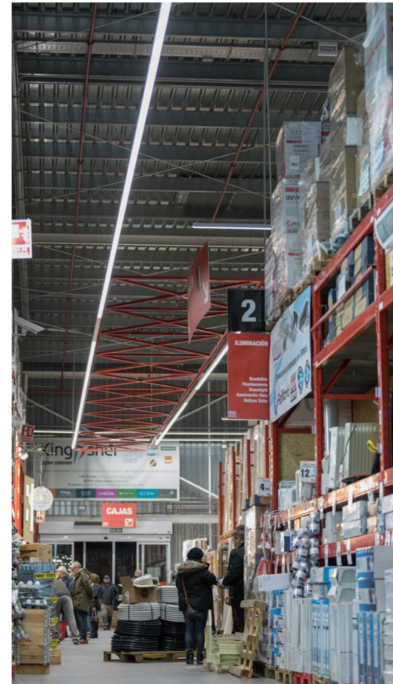
Image 1: The LED panels fit seamlessly together to create a truly continuous line of light.
